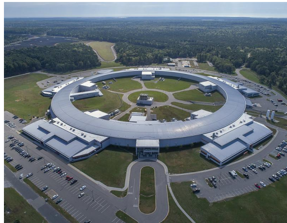
National Synchrotron Light Source II (NSLS-II) at BNL.
